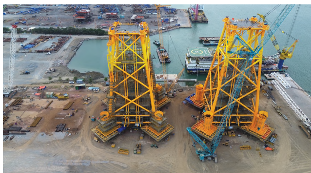
Figure 14. OWE project in a fabrication yard of a subsidiary of Petrovietnam.
